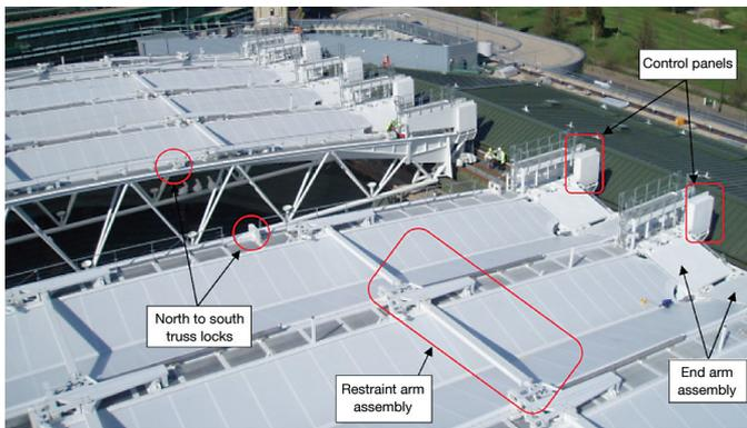
The roof deploys one truss at a time on both the north and south sections. The truss is deployed by the bogies and the end arm assemblies. The end arm assemblies look like giant inverted hinges, which open up from a very deep, narrow "V" into a wide, shallow "V".
