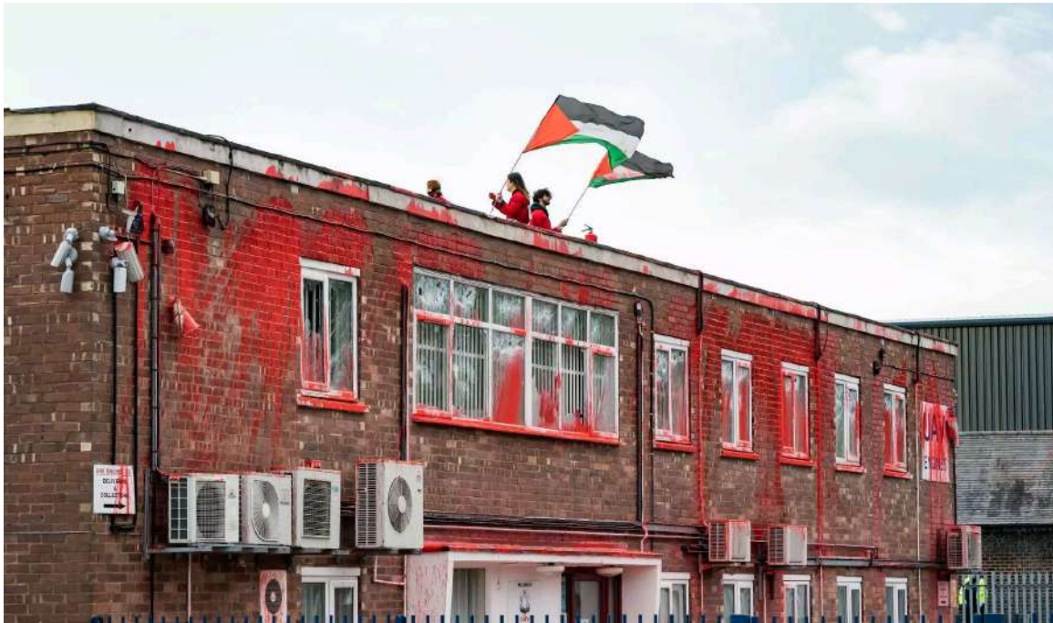
Activists on the roof of the UAV Engines factory in 2021. (Photo: Vladimir Morozov / Alamy)
