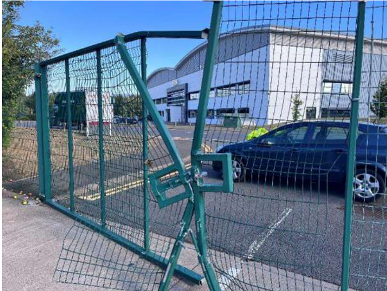
Logistics Gate (photos taken after gate made safe/secure)
